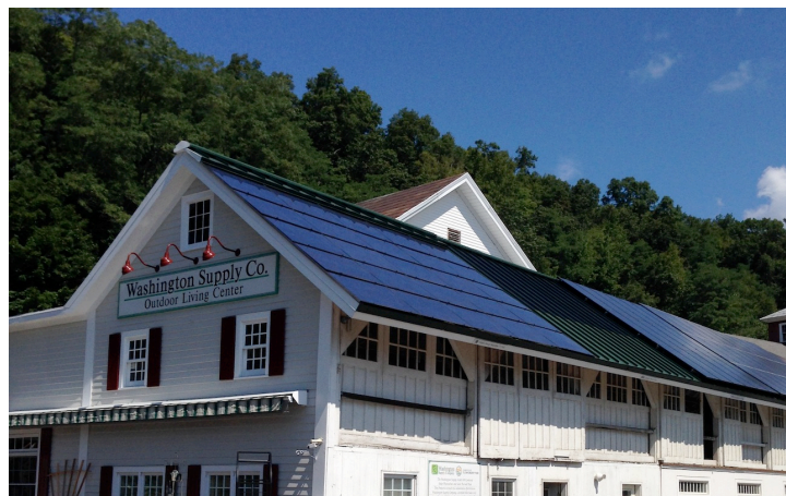
Solar Panels in Washington Depot
