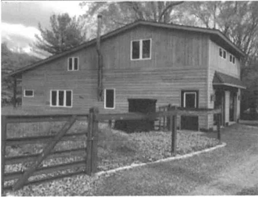
Garage prior to the fire.
