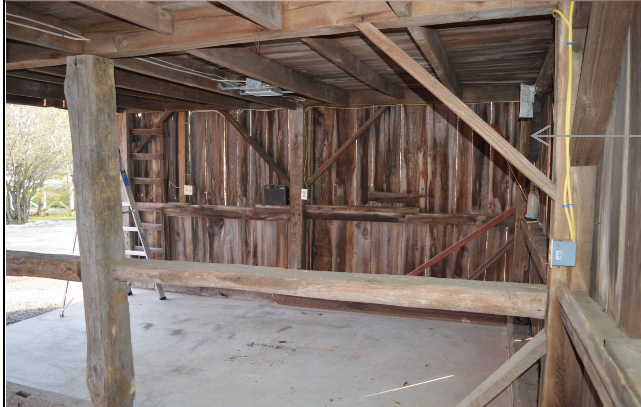
Open to weather at all times, wood is rotted in many locations.
