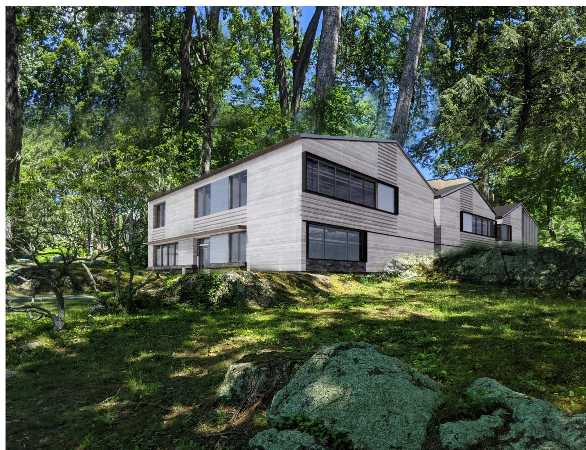
2. SOUTH EAST FACADES VIEW
